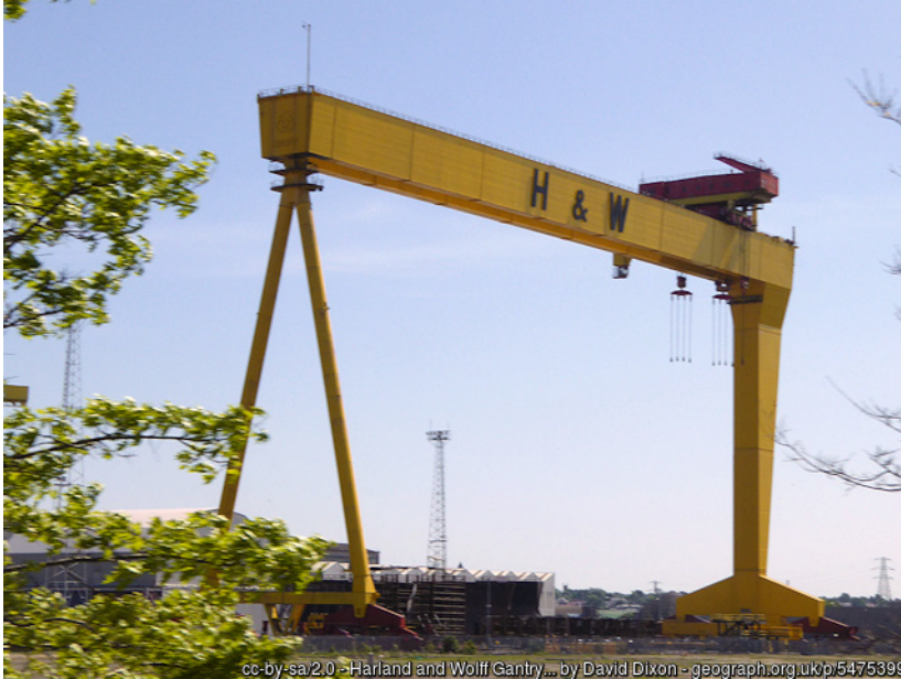
Figure 1: The Goliath crane in the shipyard of Harland & Wolff in Belfast.
