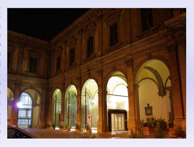
The access to the new first aid, located in the west side of the lodge, the object of present study, is realized with a steel structure and glass and equipped with two portals of access to the ambulance service and transportation of sick and a pedestrians. This new hall fits into the Buontalenti's porch with respect, preservation and protection for architectural, historical feature and cultural value of the building
