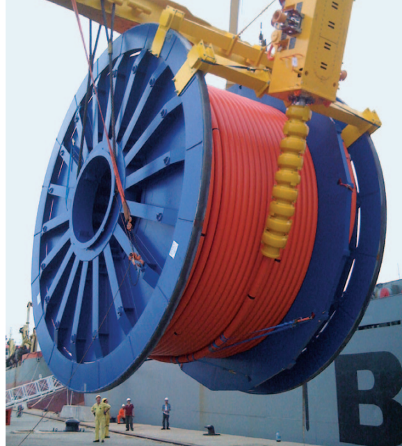
An umbilical cable on a drum ready to be placed on a ship for laying.
