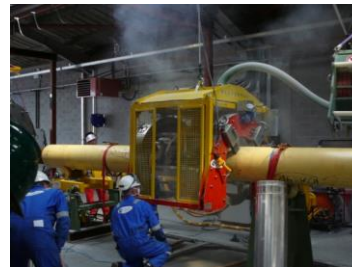
FBE application Corrosive protection
