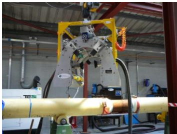
Surface cleaning Grit blasting
