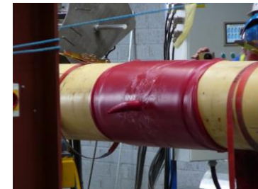
Field joint Needs cooling
